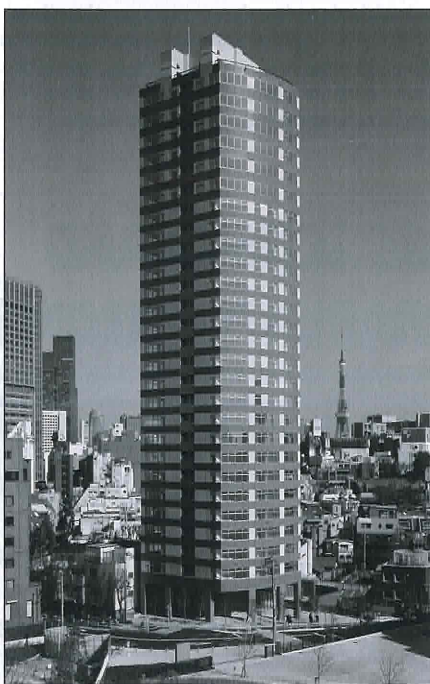
Figure 2. The Glorio Tower Roppongi high-rise residential building, located in central Tokyo, which uses ECC coupling beams in its core for seismic resistance. The building is 27 stories (95 m) high. Built by Kajima Corp., construction on the building was completed in 2005.
