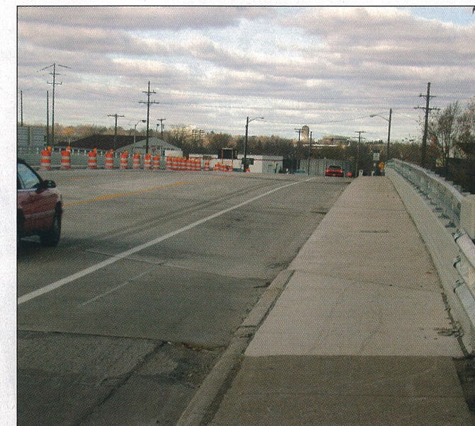
Above: A mix design for ECC and regular concrete. In ECC, there are no coarse aggregates. Instead, very fine sand, fly ash, and microfibers are included. Right: Constructed in 2005, the ECC deck link-slab on the Grove Street Bridge in Ypsilanti, Mich., eliminates frequent maintenance of common expansion joints.
