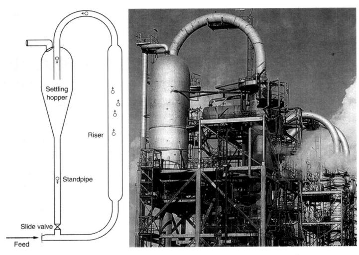
The reactor is 3.5 m in diameter and 38 m tall. [Schematic and photo courtesy of Sasol/Sastech PT Limited.]
