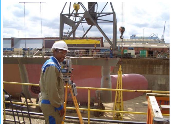
This picture illustrates cranes maneuvering a grand block for final erection
