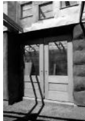
Figure 73: Refinished salvaged doors.
