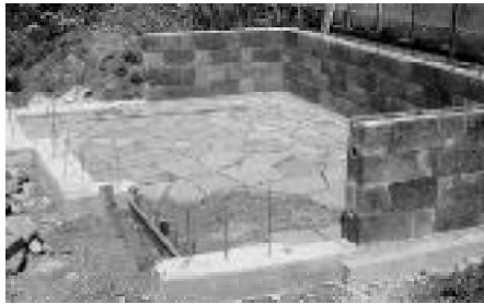
Figure 71: Setting floor “pavers” and Faswall blocks . . .
