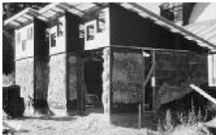
. . . and strawbale infill and Faswall waiting for stucco. The framed portion above will be sided with aluminum litho-plates.
