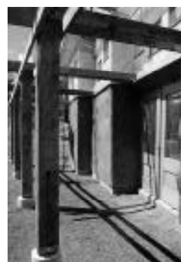
Figure 68: Exterior views of Stookey's Plant Nursery in Moscow, Idaho.
